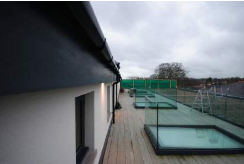
Area B: existing outdoor area enclosed by balustrade but not authorised for outdoor dining Facing South (with mocked up 1.8m screen in place)
